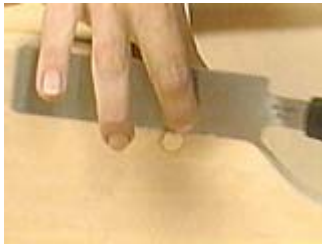
Cut off the plugs with a flush cut saw
