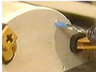
Drill the plug hole about three-eighths of an inch deep
